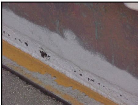
The LRUT probe pushed the sound through with the aid of thick couplant layer despite of corrosion pitting on the annular ring.
